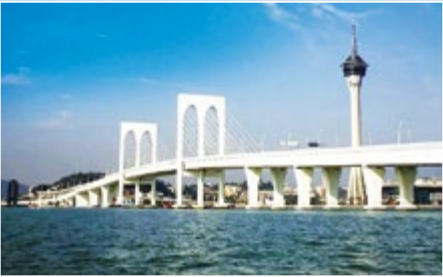
世界建築史上首創上下雙層行車道混凝土梁斜拉橋 ——西灣大橋 Sai Wan Bridge in Macao - the first innovative cable-stayed bridge providing carriageways on top of and inside the concrete box girder
