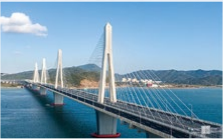
世界首座公鐵同層多塔斜拉橋、世界最寬公鐵兩用多塔斜拉橋 ——珠海西江公鐵大橋 Zhuhai Xijiang Rail-cum-Road Bridge - The world's first and widest multi-pylon cable-stayed bridge with highway and railway on the same deck.
