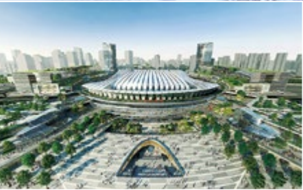
大灣區最大的火車站綜合樞紐 ——廣州白雲站 Guangzhou Baiyun Railway Station - the largest comprehensive railway hub in the Greater Bay Area
