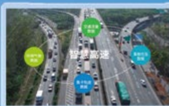
上海G15智慧高速改扩建 一体化运营示范工程 Demonstration Project of Integrated Operation for Renovation & Expansion of Shanghai G15 Smart Expressway
