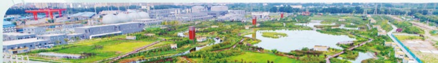
Beijing Huaifang Water Reclamation Plant / 北京槐房再生水厂
